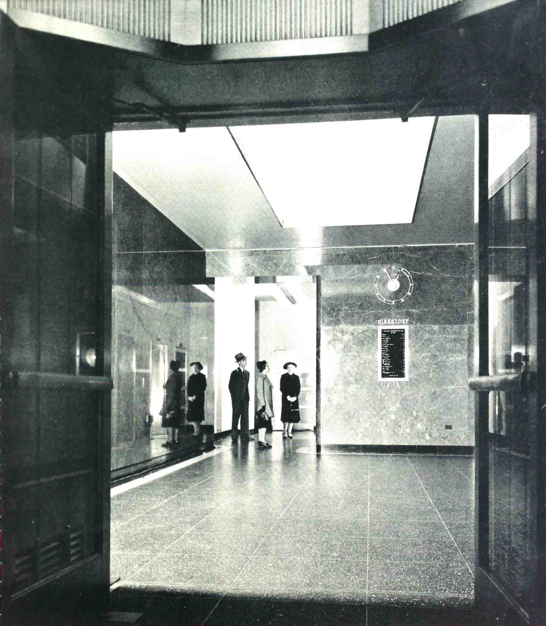
KYW's hospitable lobby in gleaming Spanish marble with bright accents of aluminum trim
